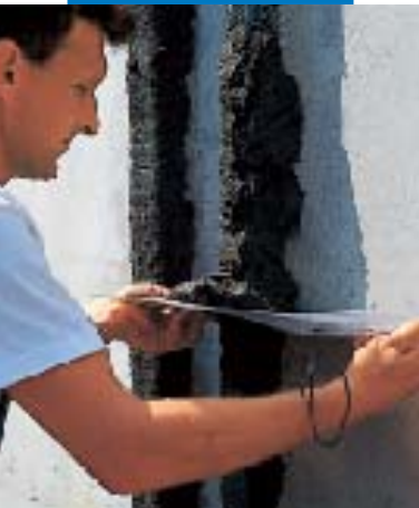
Shaping the screed
